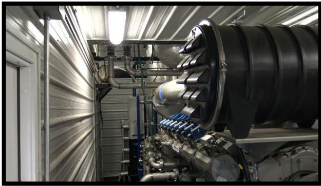
j.) 16 cylinder biogas engine
